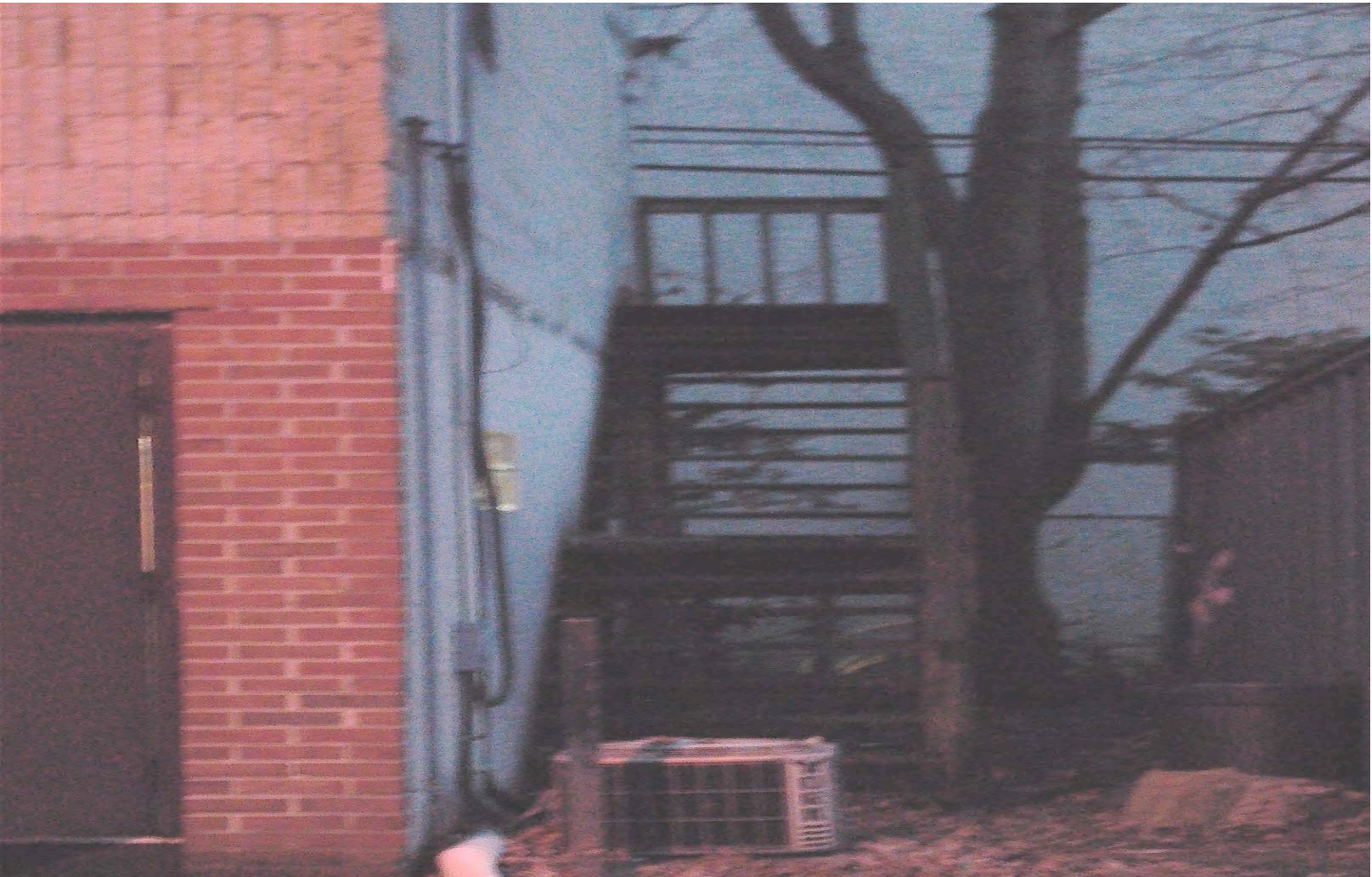
REAR EXIT AND FIRE ESCAPE
